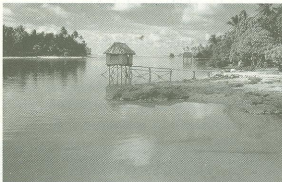
One approach was to have small 'houses' out over the water so the tide carried away the waste,
