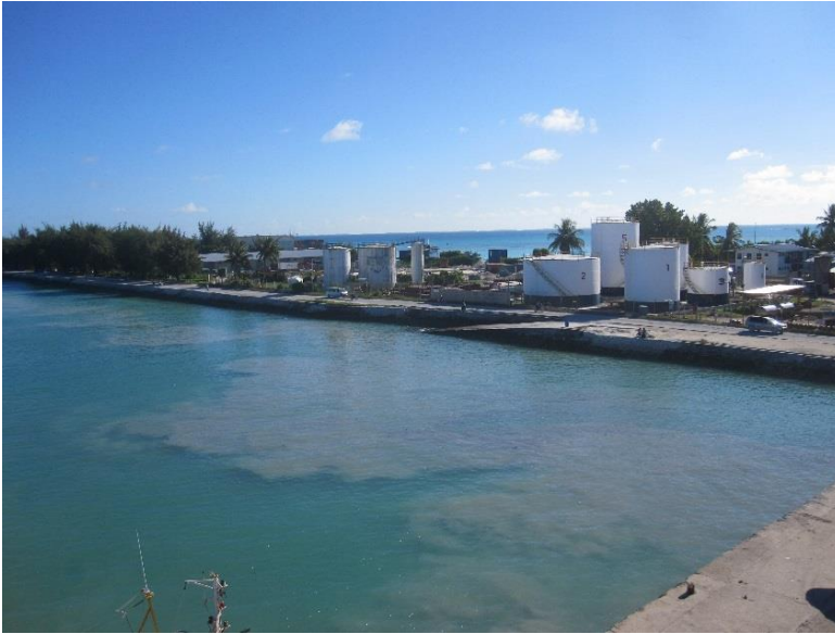
Photo 13: from crane to yards 2 & 3.
