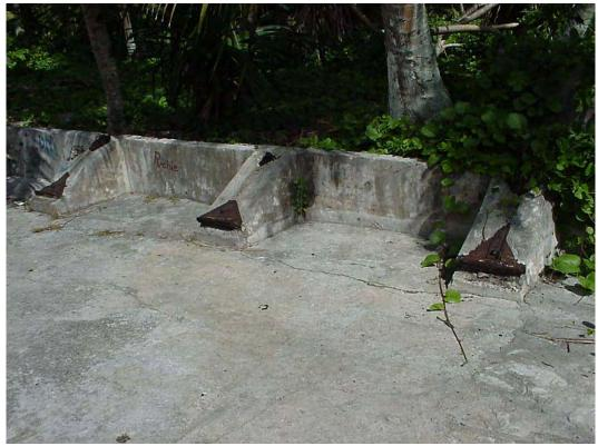
Photo 81 Hangar Wall and Roof foundation.
