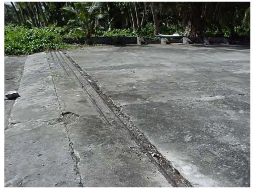
Photo 80 Hangar (rails for sliding doors).
