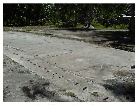
Photo 57 Hangar foundation and drainage.
