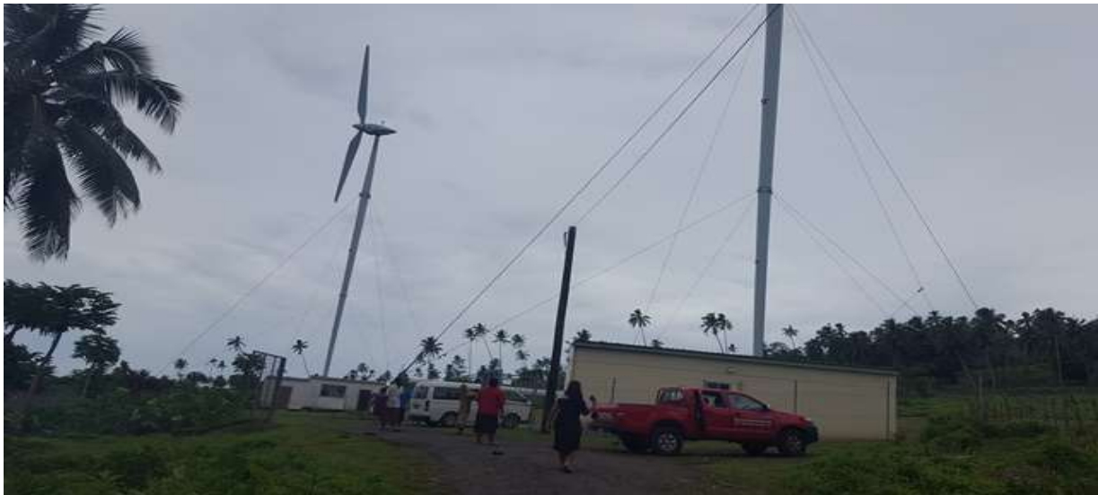
EPC Windmill Station in Vailoa and village request to reseal road to this station for easy access.
