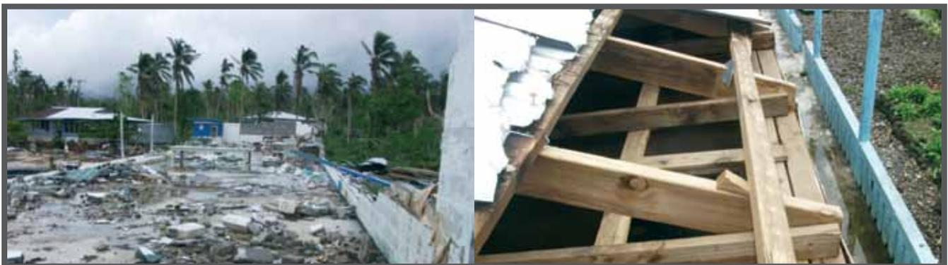
**Photos** Left: Salamumu Primary School, total rebuild required from foundations up. Right: Faleseela Primary School, Strengthening required for roof structure tie downs. Courtesy of GoS/PDNA Assessment team.
