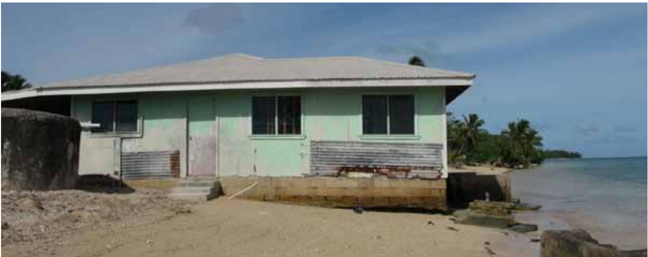
Figure 3: A house that is inundated by waves at high tide
