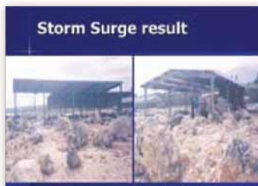
Photo12: Strong storm surge damaging Nafanua Harbour, MoW, 2003.
