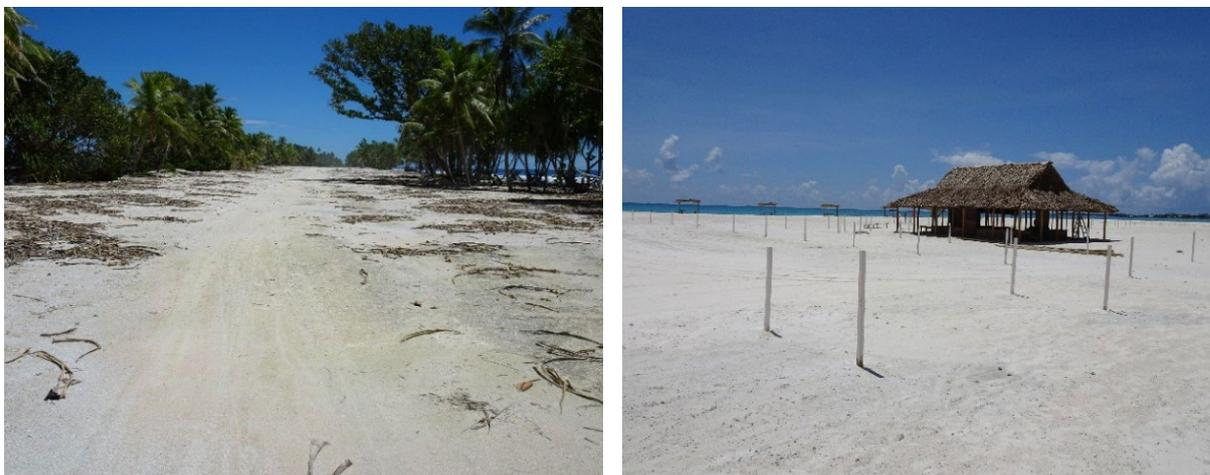
Figure 6. Former borrow pits north of the garbage dump reclaimed in 2014 and infilled with lagoon sediment dredged from Funafuti Lagoon (left); and the extensive reclaimed area on the lagoon side of the Tuvalu Government Building and Vaiaku Lagi Hotel, which was formerly opened as Queen Elizabeth II Park in early 2016 (Source: Thaman 2016).
