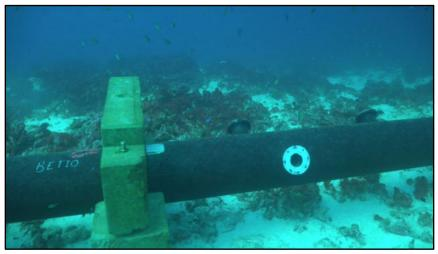
Figure 11 – Photo of outfall opening with diffuser ports, Betio (30 m depth)
