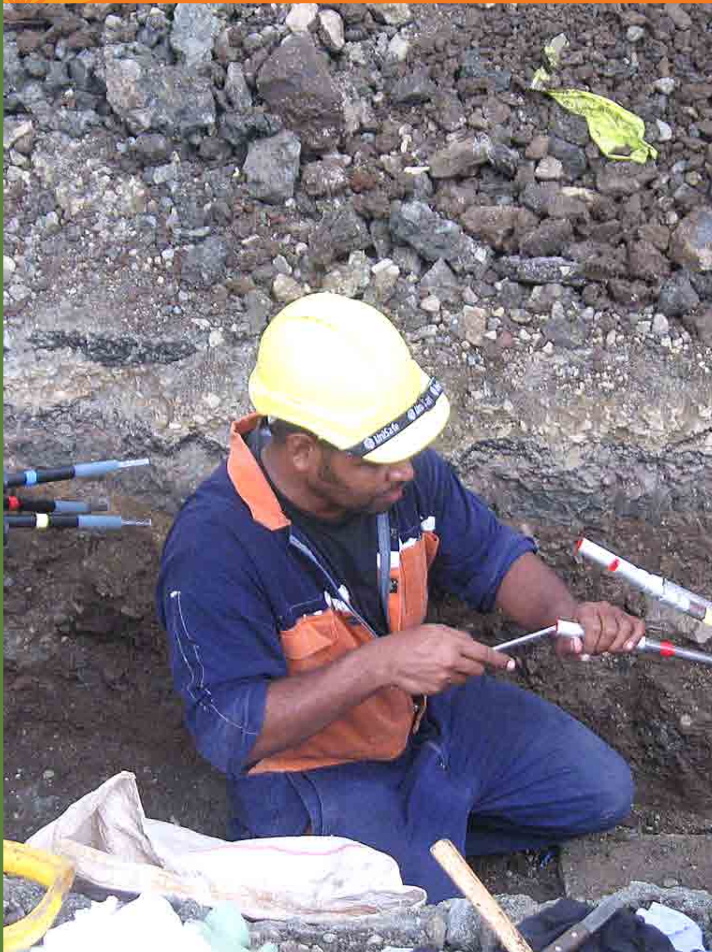
FEA employees work continuously around the clock to ensure minimum power disruptions to customers. An FEA tradesman is seen here repairing a faulty underground cable.
