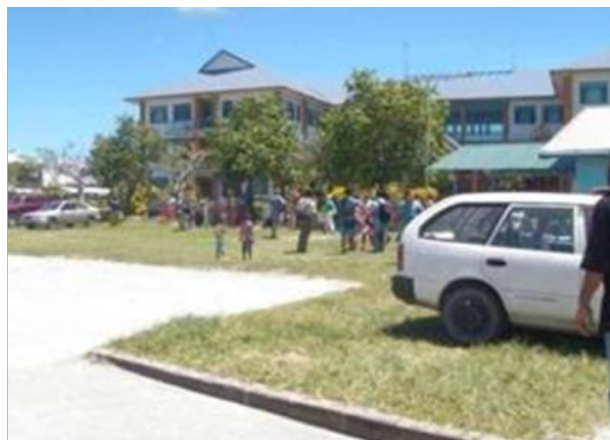
Government Building in Funafuti
