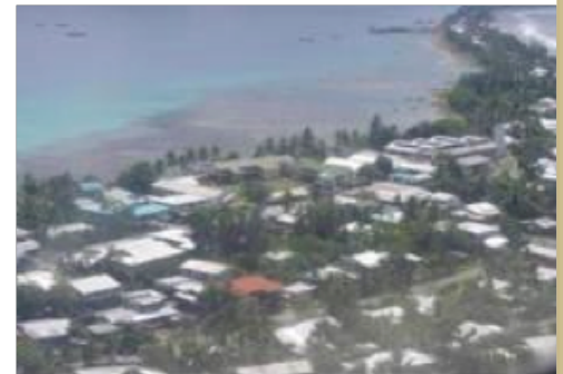
Potential "solar roofs" in Funafuti
