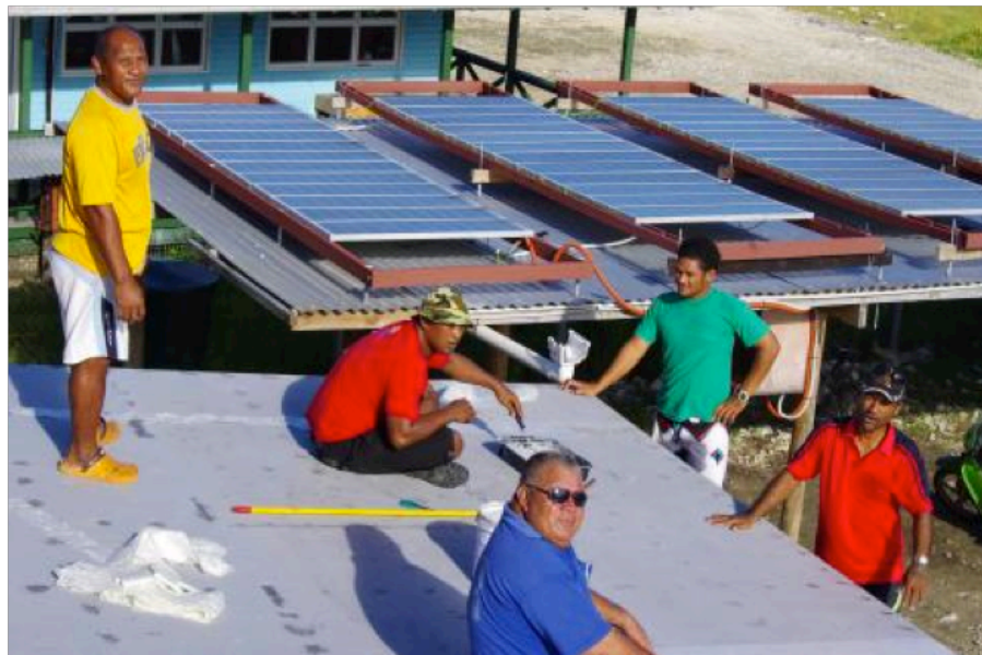
TEC staff installing a non-metallic, low maintenance and cyclone proof demonstration solar roof
