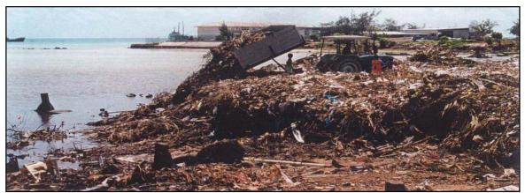
Fig 3. Landfill at Betio before SAPHE Project (no proper containment (SOER 2000-2002)
