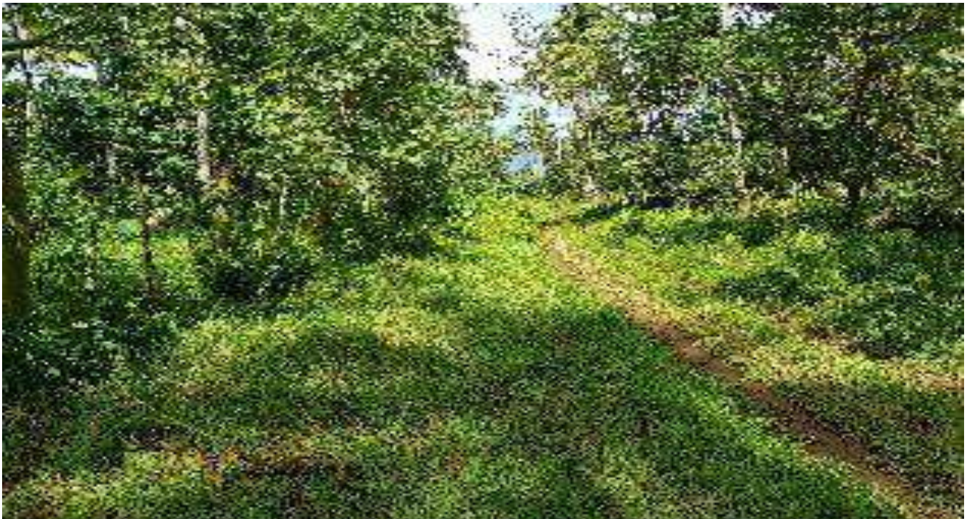
Access Road to Plantation in Vavau request tar sealing
