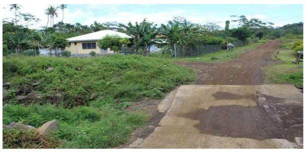
Ford at Moamoa-fou towards Catholic Resettlement Area, when it is heavy rain and flooding it will stop vehicles from crossing and can isolate families on the other side of the ford with no access to cross if there is an emergency. Long term solution is replace ford with a bridge
