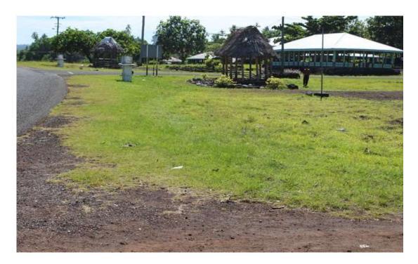
Sasina Village main road - has no road side drainage and prone to flooding.
