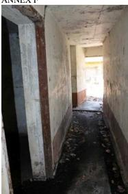
Figure 20 Bunker interior - note good paint condition and loss of wood door surrounds.
