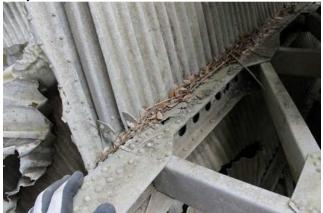
Figure 7 Corrosion is higher where debris can trap water.
