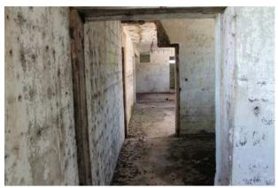
Figure 25 Interior of main observation complex. Note that all wood has been eaten by white ants and rotted completely causing some losses where it was structural.
