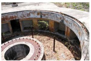
Figure 5 Gun emplacement note damage by plant growth and lack of damage by corrosion.
