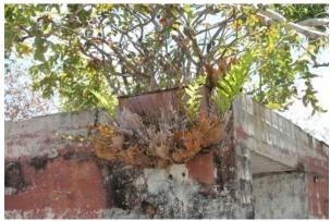
Figure 24 Plant damage to building
