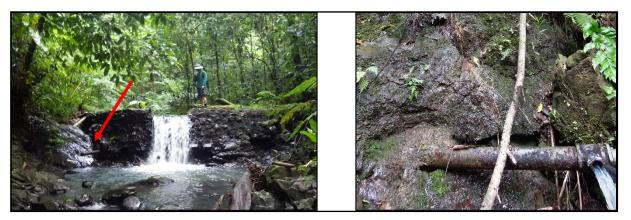
Figure 15: Example photos of village water system intakes. Abandoned village water impoundment across Fagaalu stream (left). Note old delivery pipe as indicated by red arrow. Village water intake located directly in volcanic spring in rock face of cliff in a village near Nuuli Village (right)
