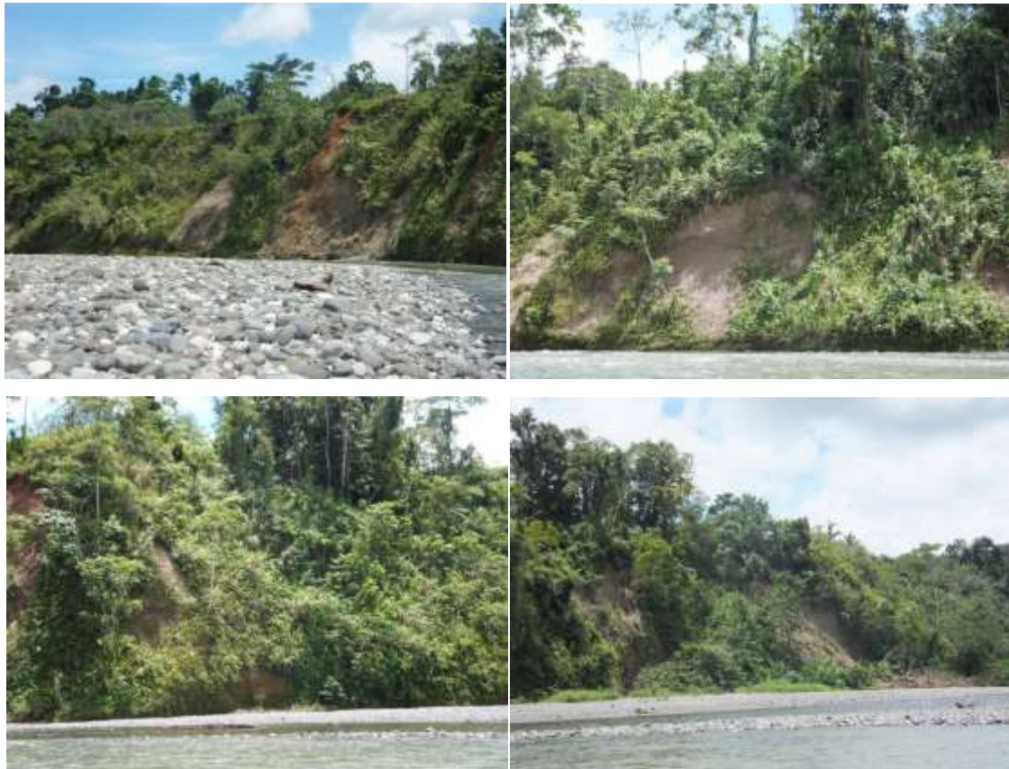
Figure 14-4 Landslides on Ngalimbiu near confluence of Tina and Toni rivers
