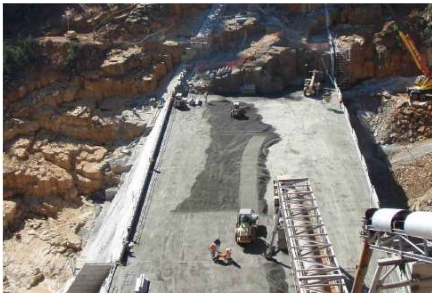
Figure 0-5 Example of RCC Dam Construction
