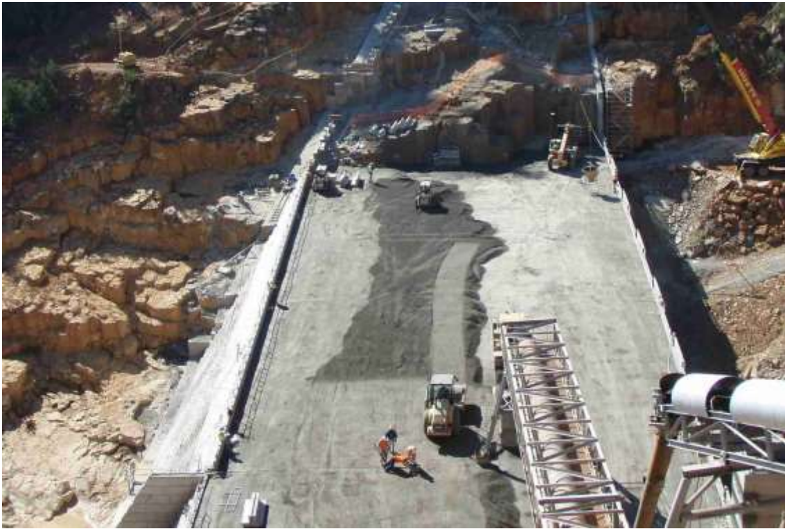
Figure 2-5 Typical RCC dam construction with concrete conveyor
