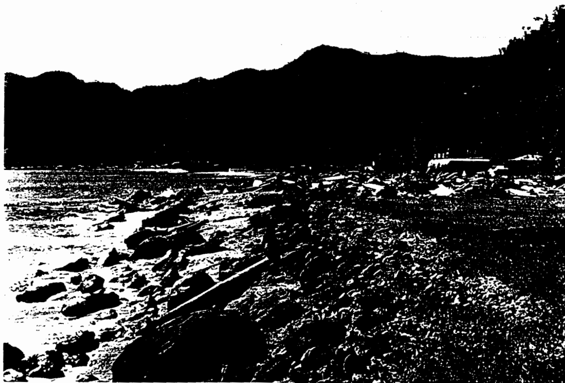
Plate A4. Shoreline of the sanitary landfill reclaimed land showing loosely-placed boulders and erosion of the upper seaward edge. View to the north.
