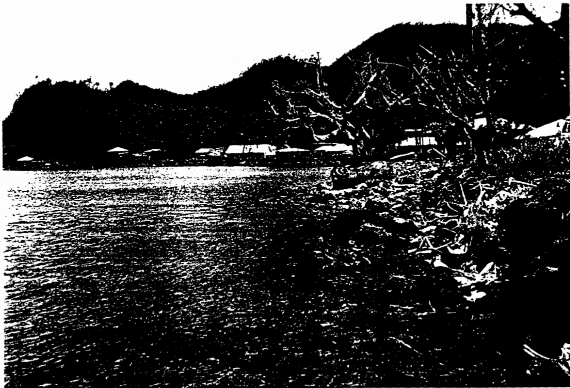
Plate A7. Shoreline within Fagaitua Bay showing loosely placed basalt boulders on the seaward side of the road.
