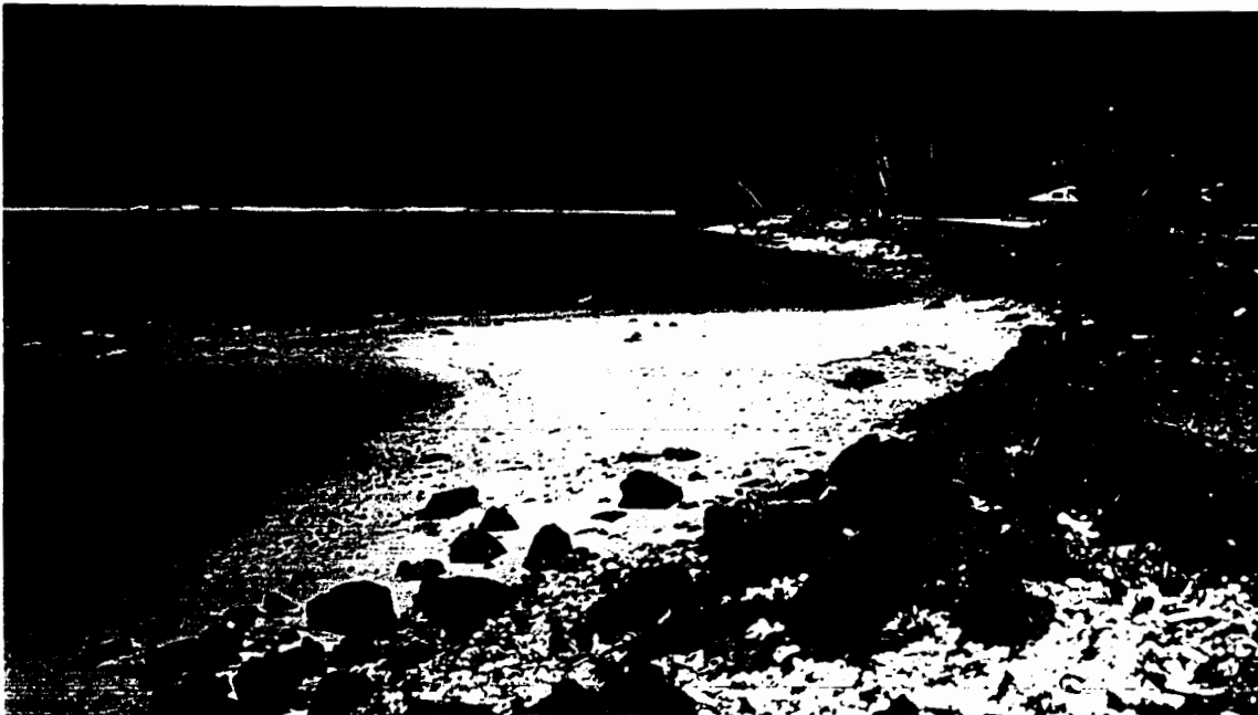
Plate A6. Shoreline near Auto showing basalt boulder revetment to stabilize the coast road and an accumulation of carbonate sand on the reef flat. Only small areas of beach remain.
