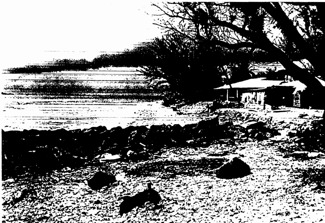
Plate A11. Shoreline of western 'Aunu'u showing a small groin of basalt boulders constructed as a result of erosion associated with the small boat harbor.
