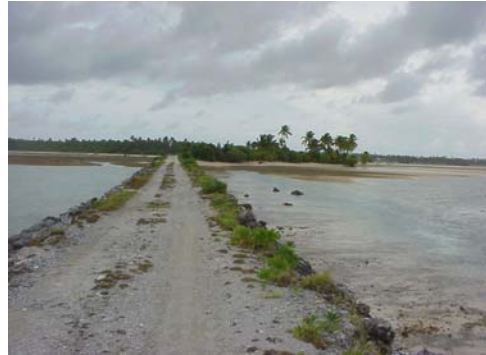
Causeways reduce seawater flushing of lagoon.
